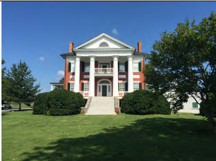
Figure 3 – Elmwood, also known as the Hugh Caperton House, is a historic home located near Union, Monroe County, West Virginia. It was built in the 1830s, and is a two-story, nearly square brick dwelling with Greek Revival details. The front facade features wide limestone steps and a veranda, with second-story balcony, Chinese Chippendale railings at both levels, and four plain but huge plaster covered brick columns. The house was built by Congressman Hugh Caperton (1781–1847). It was home to Allen T. Caperton (1810–1876), the first ex-Confederate elected to the United States Senate after the American Civil War. - Wikipedia
